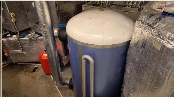
Bilete 21 – Akkumulator tank for kjølevatn (1000 liter).
